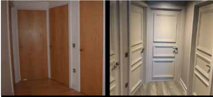
We modernised this hallway by changing the flooring and having moulding added to the original doors and having them spray painted in a factory to get a perfect finish before adding new door furniture.
